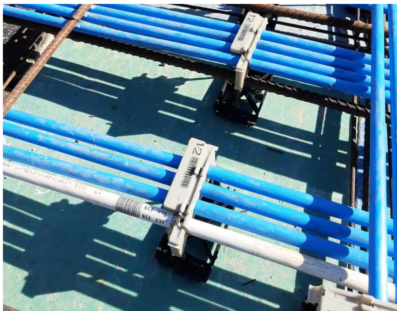
Figure 84: Bundle fixed by the tendons grippers at the desired elevations.
