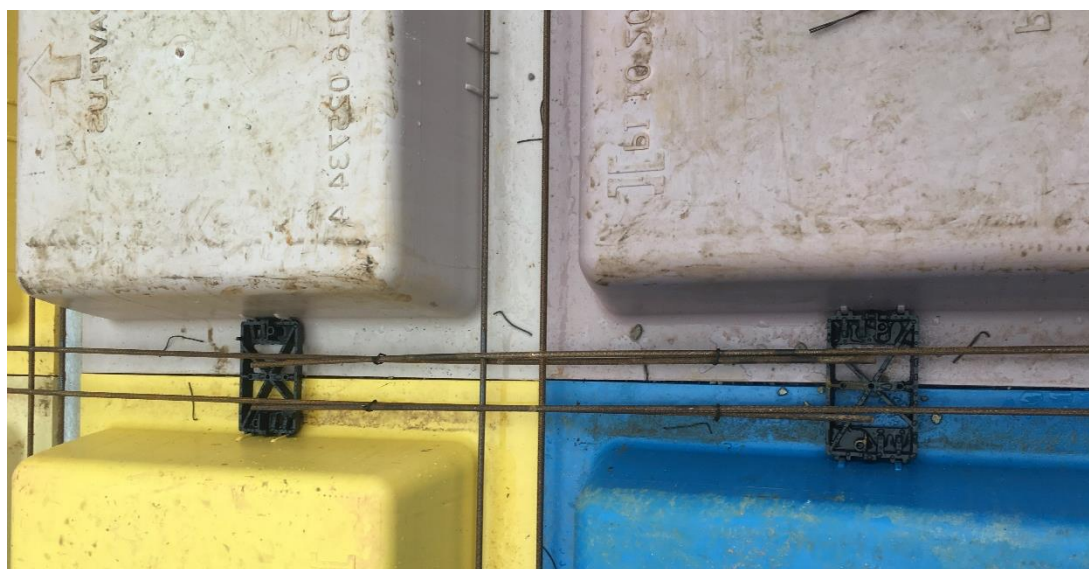
Figure 69: Barge stuck in the ribs of the waffle mold and receiving the rebars.
