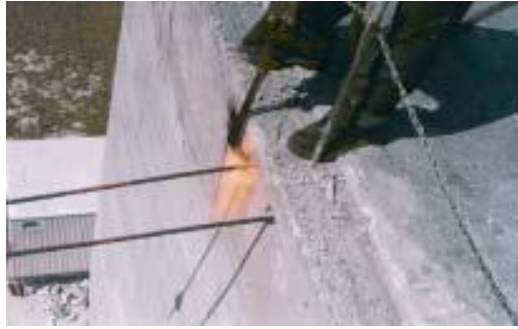
Figure 93: Tendons being cut with the aid of the blowtorch.
