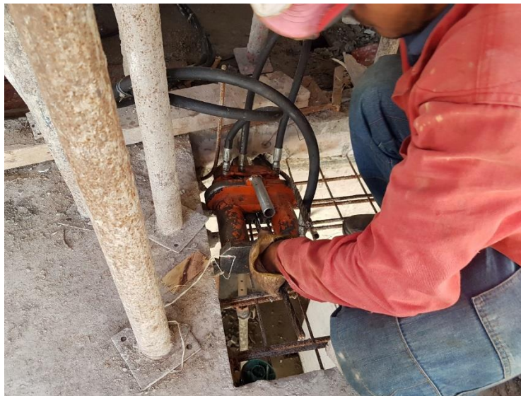
Figure 90: Fitting of the jack to the strand.
