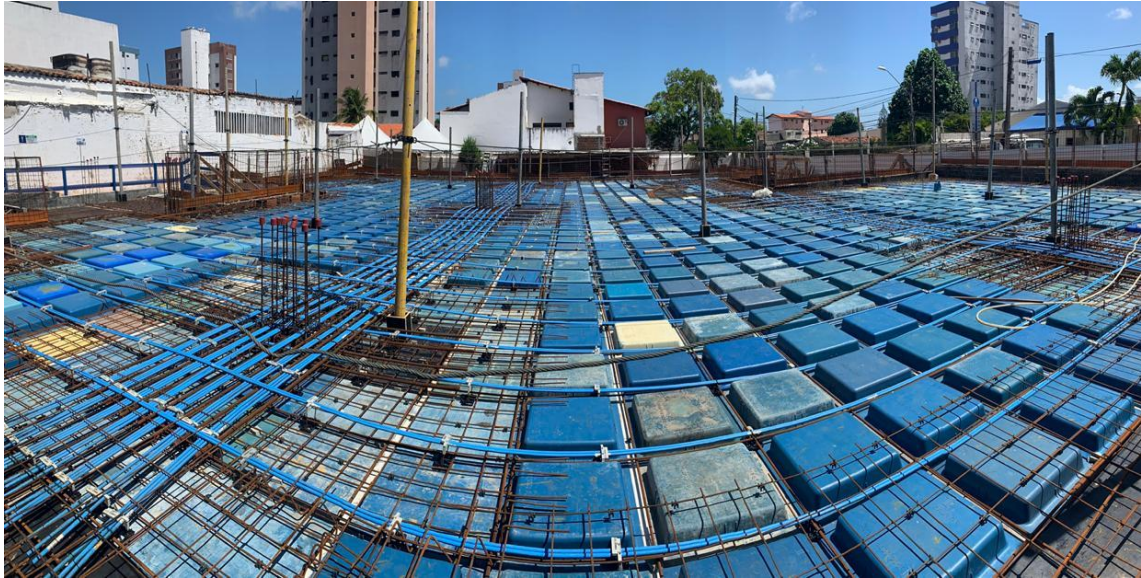
Figure 86: Completion of the assembly of the post-tensioning in the distributed regions.
