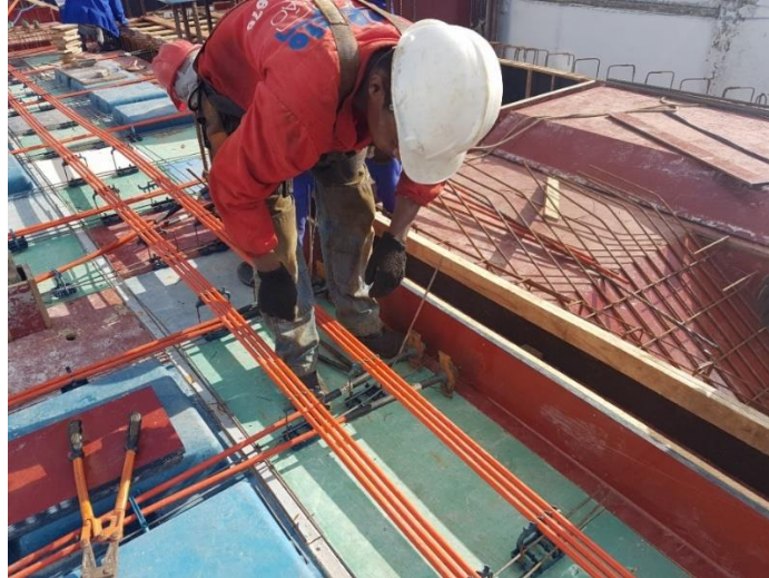
Figure 82: Dead-end anchors being fixed and aligned.
