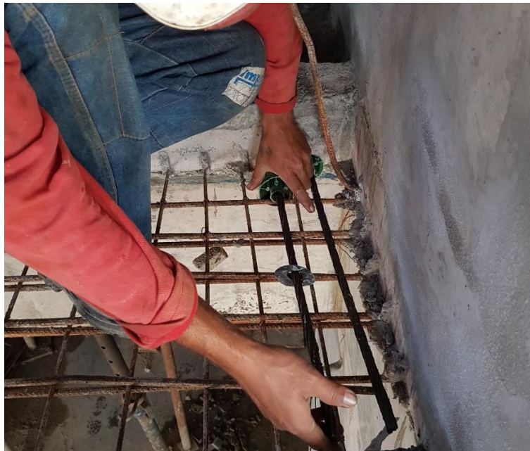
Figure 87: Pocket Forms being removed to clean the niches.
