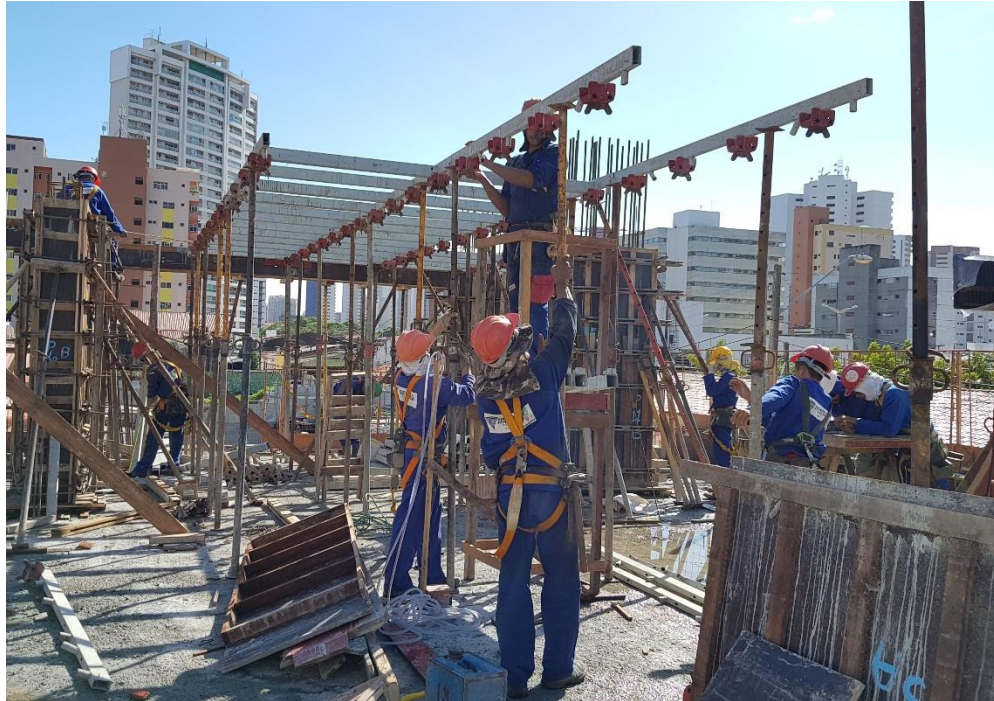
Figure 63: Suspension and stabilization of the Main Joists (LPs).
