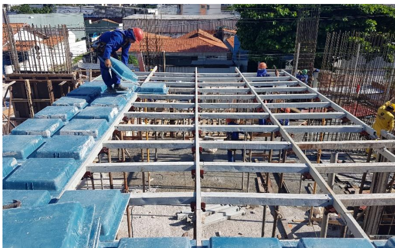
Figure 66: Unskilled labor positioning the waffle mold to the LDs.
