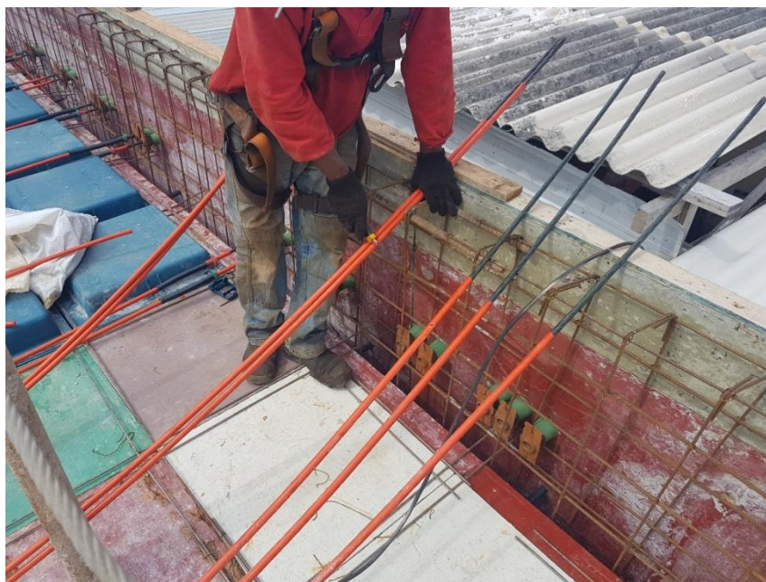
Figure 80: Tendons being cut to be positioned at the live-end anchorage.
