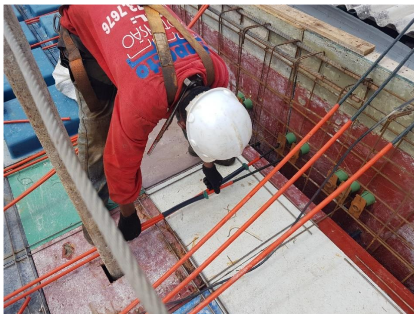
Figure 81: Tendons being positioned on live-end anchors.
