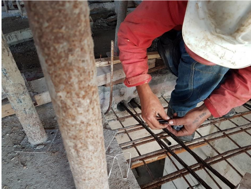
Figure 88: Wedges being positioned.
