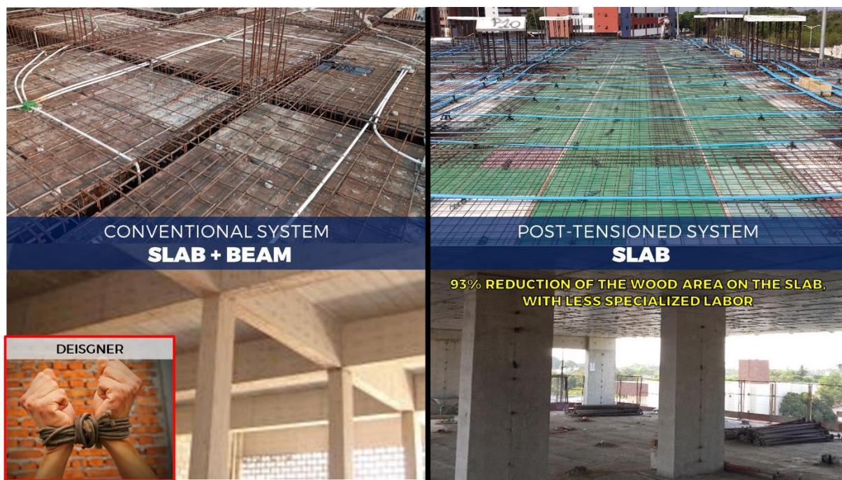
Figure 4 - Formwork systems for slabs.
